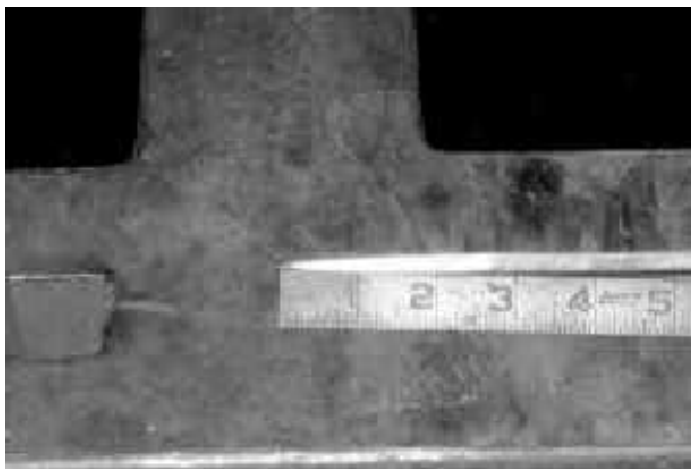
7. Side view of finished ribbon taper, and checking with straight edge.
