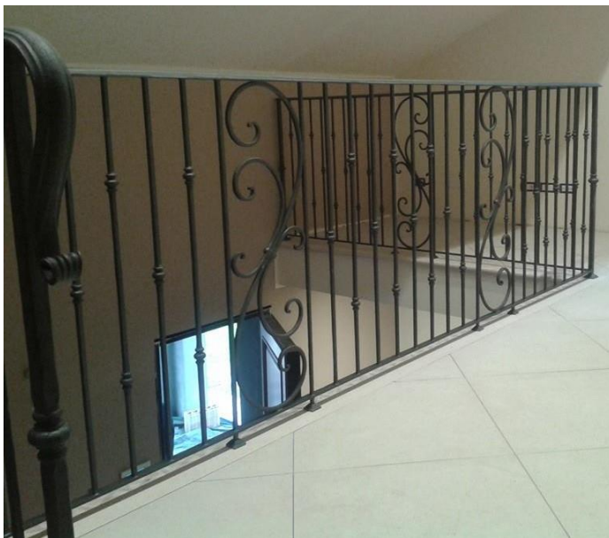
As a big fan of scrollwork, this railing has plenty of them. From the forge of Stefano Strada in Cesena, Italy comes this simply scrolled railing.
