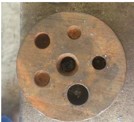
Base plate with holes drilled
