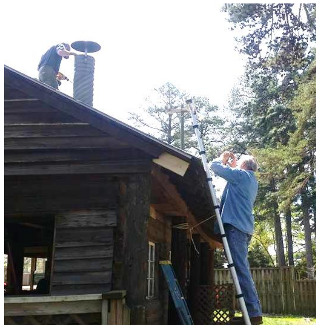
Removing the chimney
