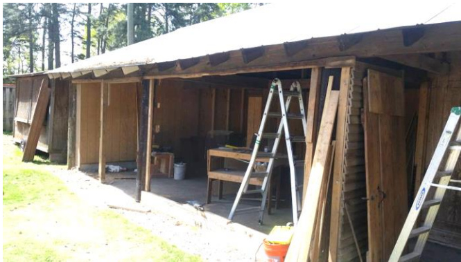
Even the walls are coming down
