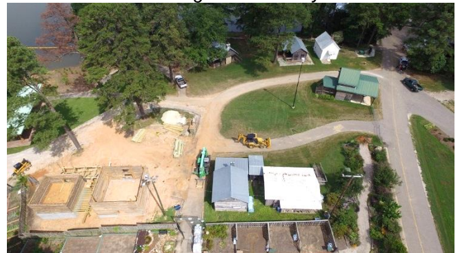
Ariel shot during construction
