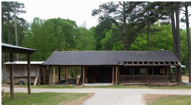
The old building waiting to be torn down.
